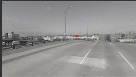
Tower Placement from Bridge (Image courtesy of google maps)
